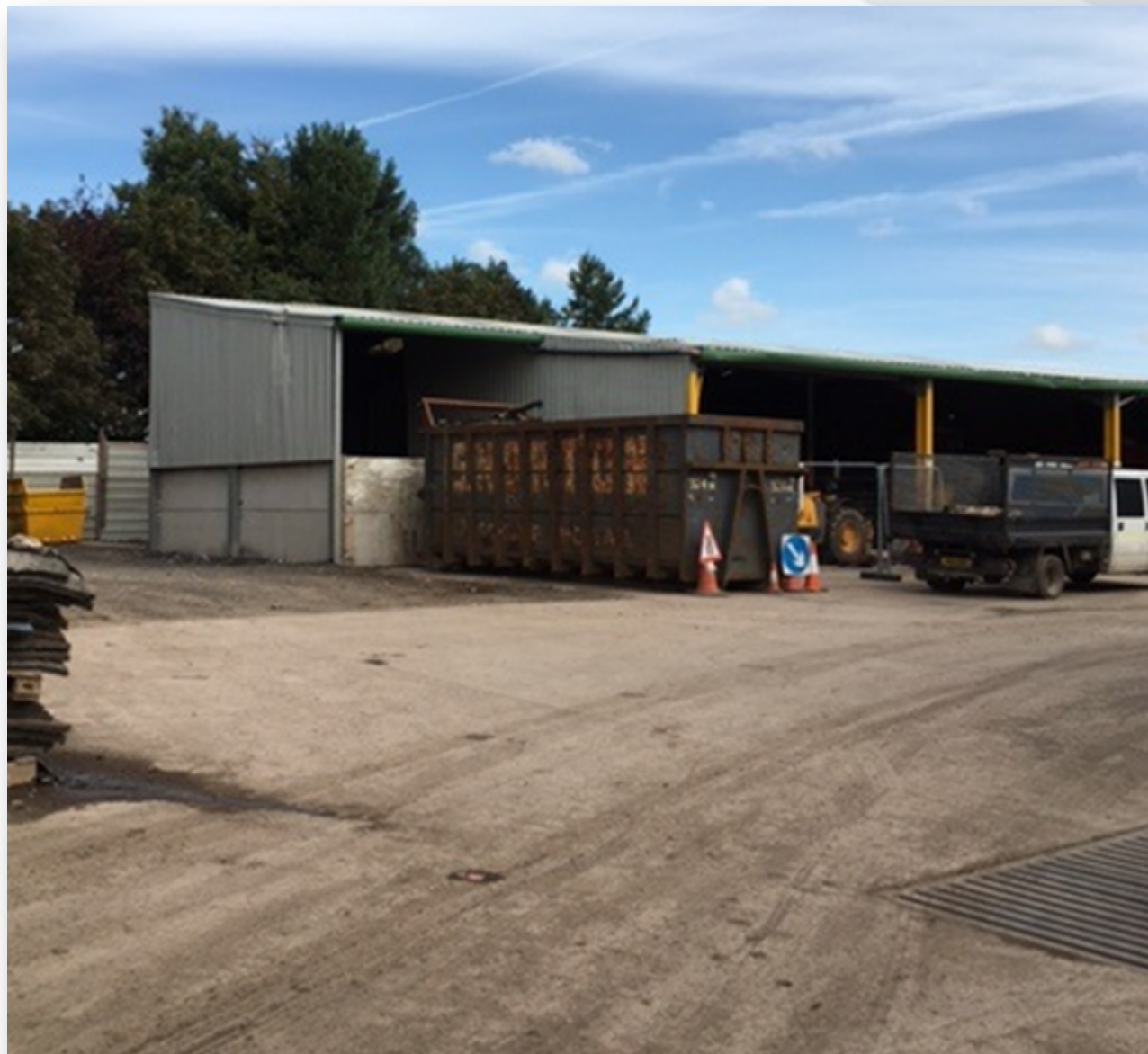
Waste management building
