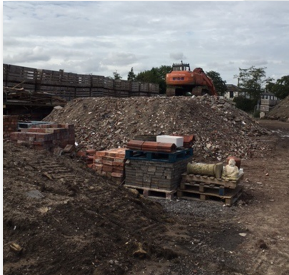
Existing outside inert storage (to be removed)
